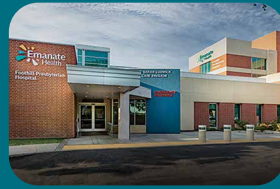
Foothill Presbyterian Hospital
